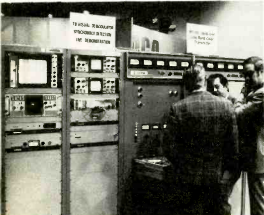
The Harris 18 kW low-band VHF transmitter. 214
