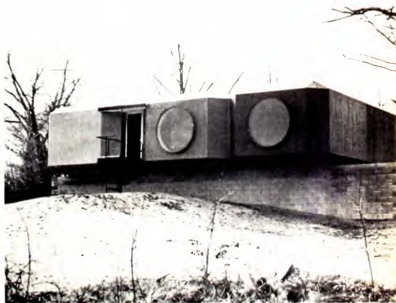
Front door of completed building is reached by open metal stairway. Sound isolation for studio is built into module. Round windows carry out architectural style.
