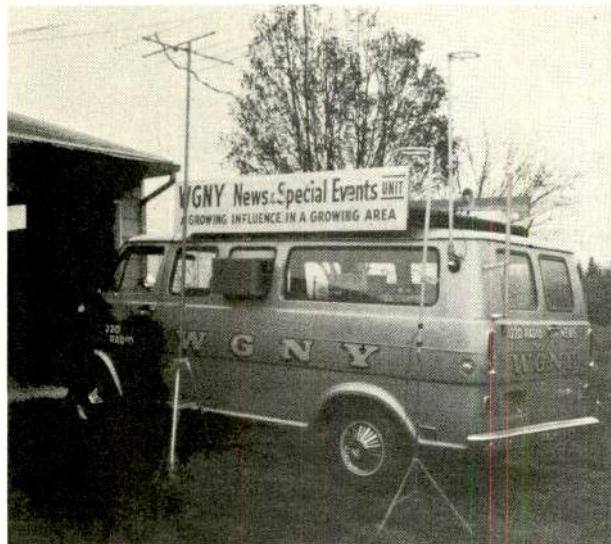
Fig. 8. Exterior view of van with various antenna mounts. Mount for yagi is on rear.
