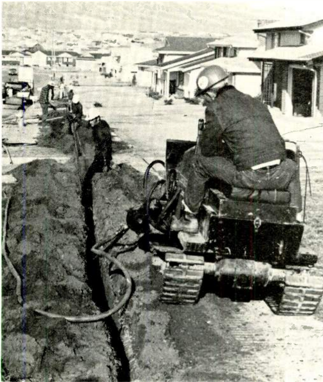
Davis Trencher is used to excavate trench in Colorado Springs residential area in Daniels cable-laying (far left). Above: Davis Hydra-Borer goes under driveways and streets. Right: Workman cleans up around trench, an important "public relations" phase.
