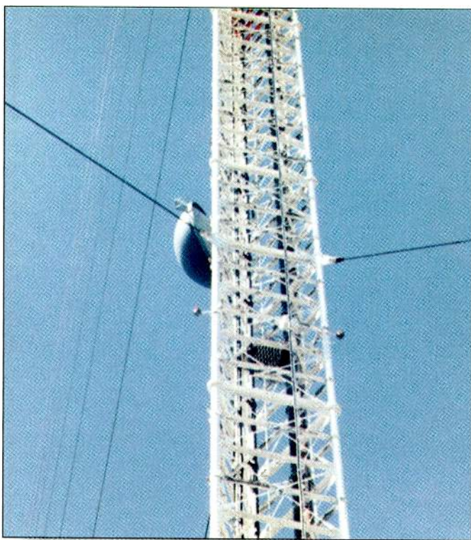
Microwave systems are common in today's television operations, with most existing systems having been in use for some time. Newer modulation schemes allow broadcasters to replace older units with systems that can transport all necessary signals.
