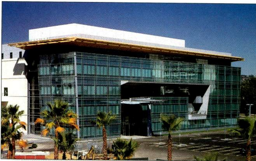
In the tapeless, totally file server-based broadcast playout center behind the new glass and polished steel, deco-styled building and the famous 20th Century Fox logo in Los Angeles, video is touched once and never tinkered with again. Fox's tapeless operation has proven to be quite cost-effective.
