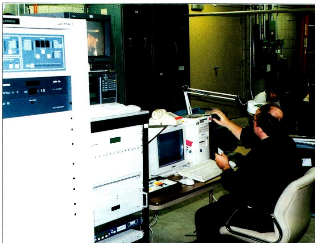
Transmitter site with the Harris 200W Ultra 1 on the left and rack-mounted Philips encoding equipment just to the right. Philips engineer Ben Sorensen configuring the Philips encoder/multiplexer.
