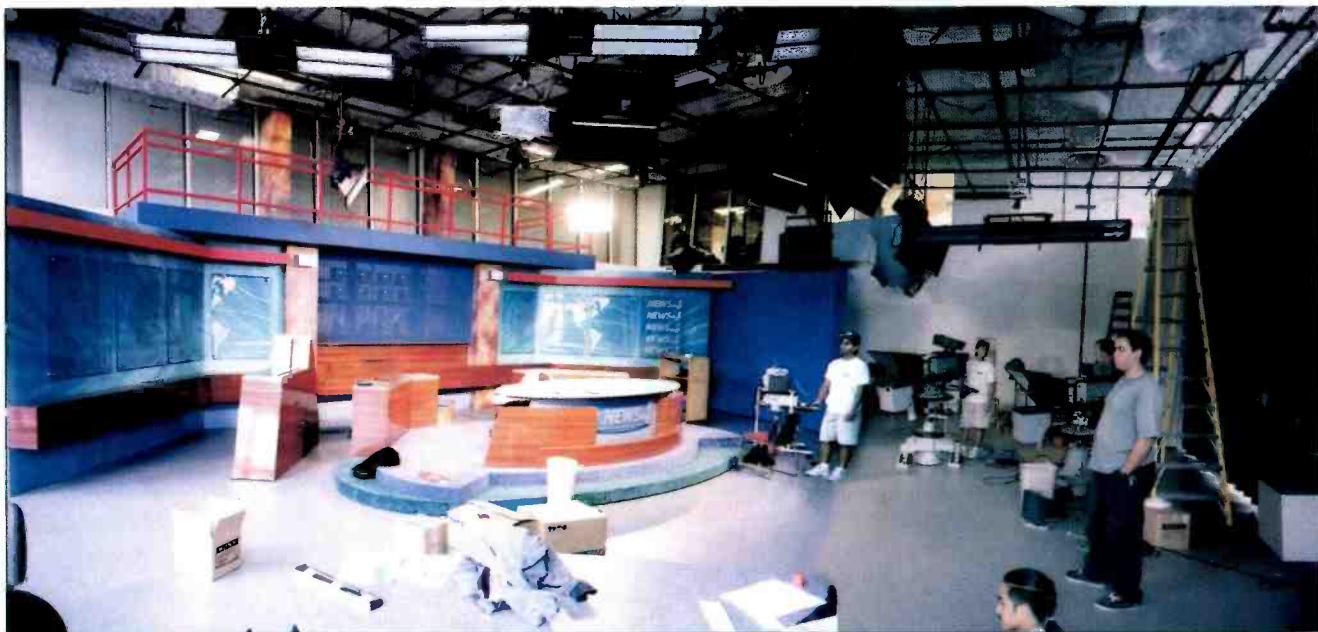
The newsroom area under construction.
