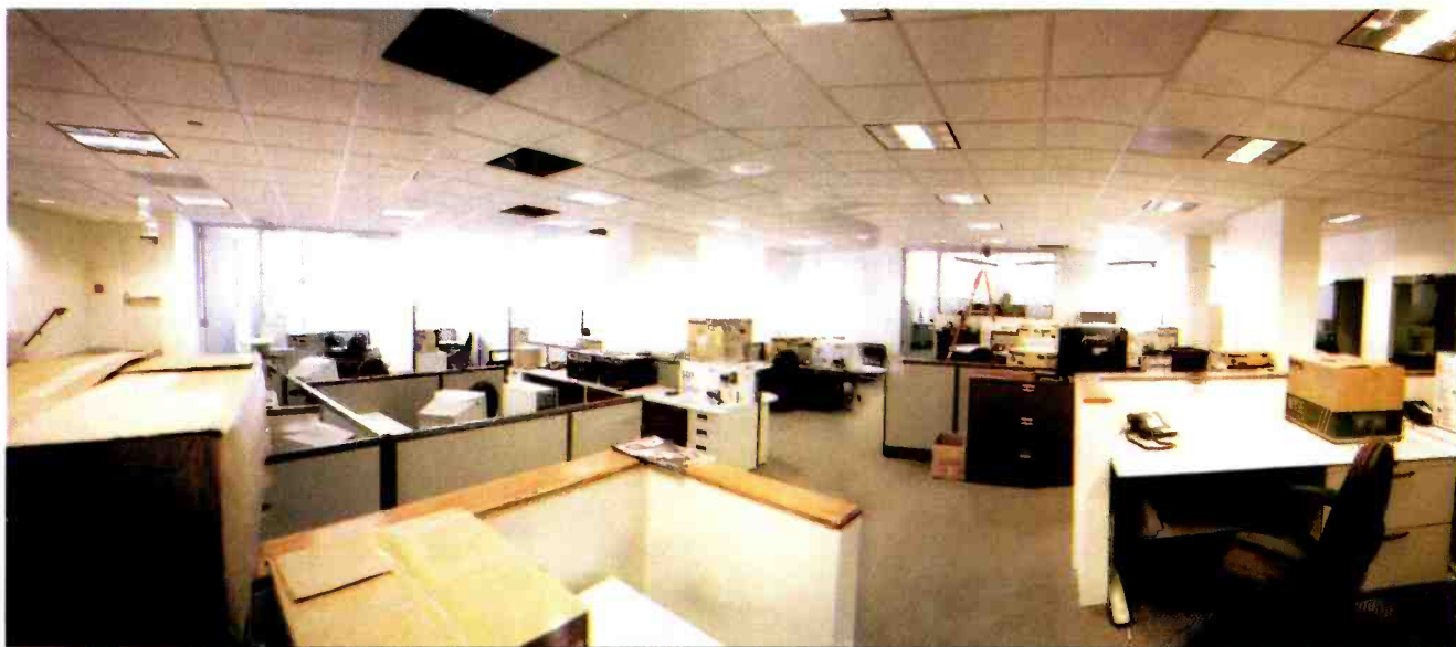
The newsroom area under construction.
