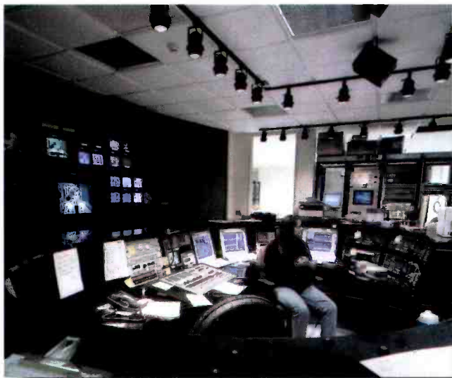
Shown on the right in the master control room are the JVC Digital S decks, the station's house format.
