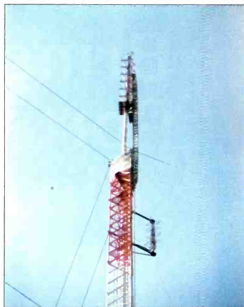
Mounting of Channel 4 WTAE antenna atop a modified TF Superturnstile antenna in Pittsburgh, PA.
