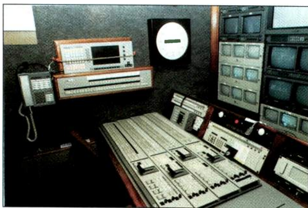
Sony's DVS-7000 switcher in LIN Productions' digital mobile unit essentially looked the same during setup as it did for the three World Series games in Atlanta. The switcher was linked with the DVS-7000 in NMT's DX-2 truck to mimic every switch for the international feed, so there was no need for a technical director at this unit during the game.
