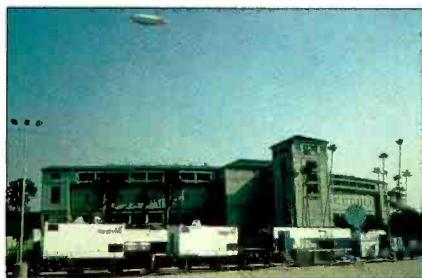
Diesel-powered generators in use in the broadcast compound at Super Bowl 1993 in Pasadena, CA. (Photo courtesy of Aggreko.)
