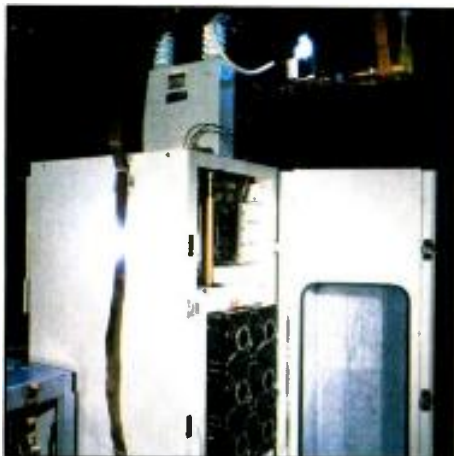
A solid-state transmitter during high-voltage discharge (lightning) testing.
