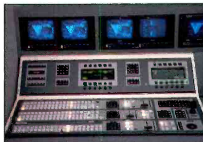
The composite video switcher at Vidcom Post, Burbank, CA. Users adjust the switcher controls with soft menu keyboards. The switcher has two M/Es.
