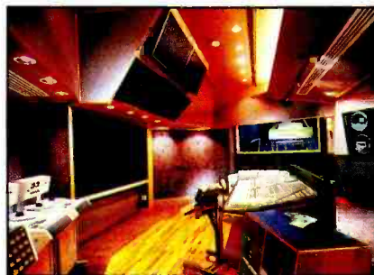
Whitney Houston's studio. Note the large expansive ceiling with special acoustic treatment directly behind the console at the listening and ceiling levels. (See Figure 2 for the floor plan and Figure 4 for the section.)
