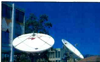
Although fiber plays a large role in how signals are handled, two dual-band TVRO dishes are required for some program acquisition.
