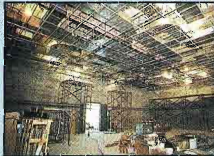
The main WJLA-TV studio during construction.
