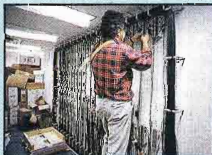
Wires, wires everywhere! A worker wires the audio punchdown blocks.
