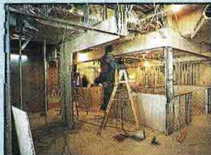
One of the edit booths during construction.
