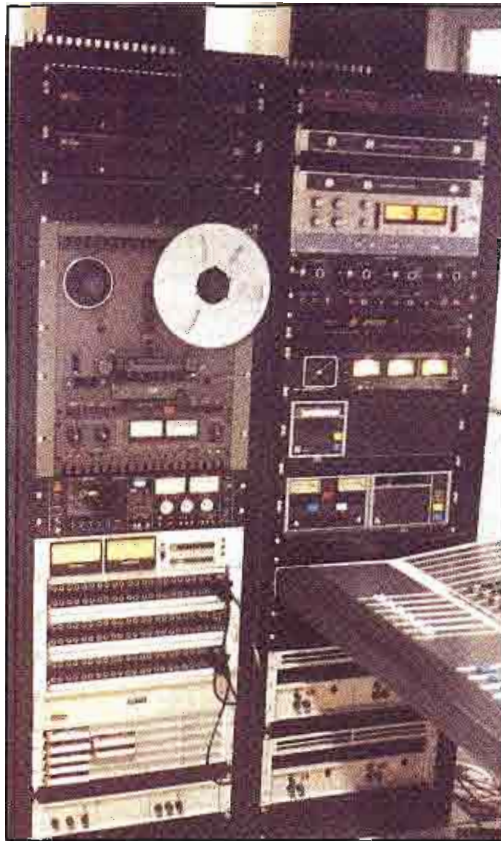
Ergonomics play an important role in the operational success of a facility. Note the easy access to audio source equipment from the audio console operator position.
