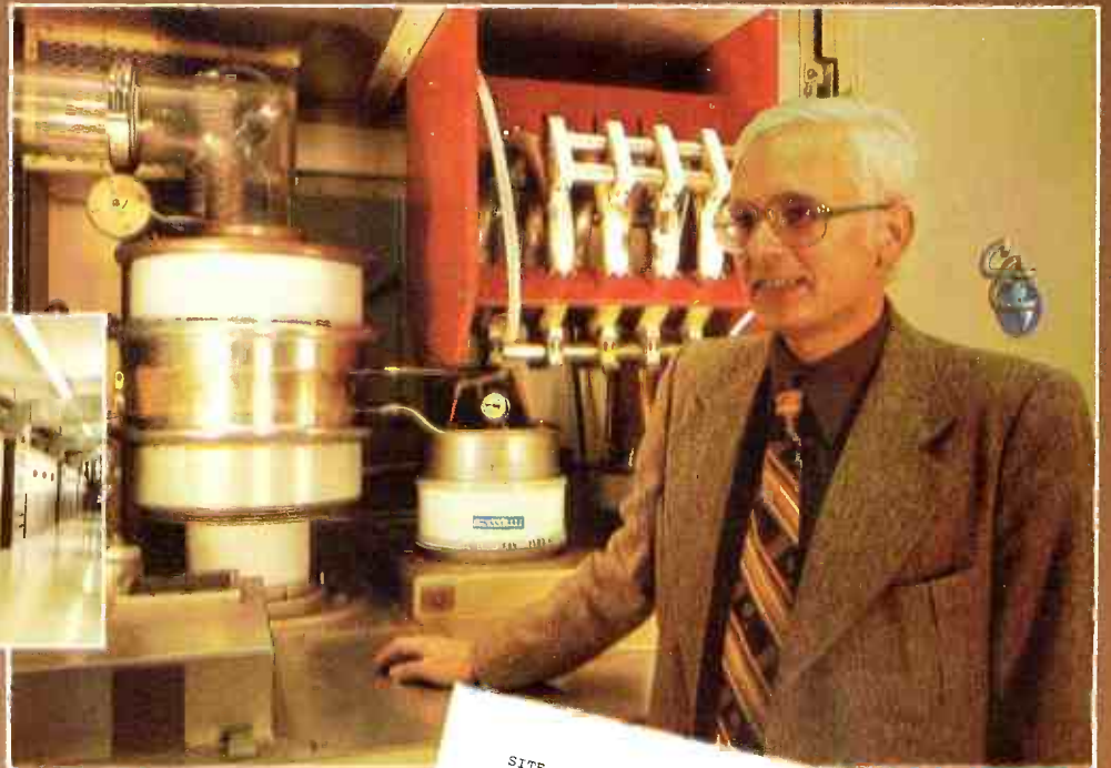
Hugh Fallis, VP Engineering, Radio Free Europe, Munich, stands beside CE 100 kW HF transmitter using EIMAC 4CV100,000C tube.
