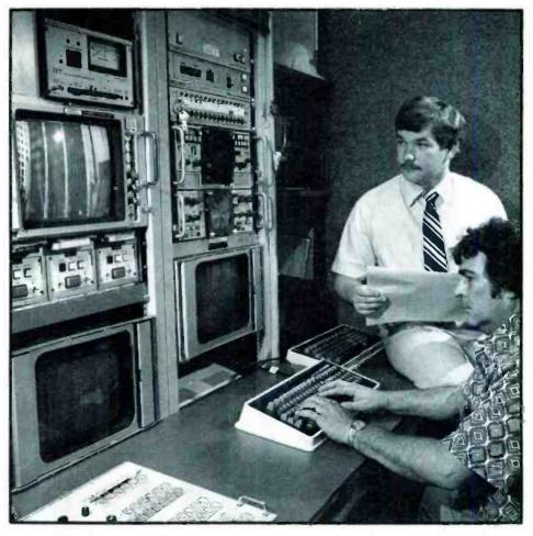
The WISH-TV automation system cuts on-air errors and improves billing. Charlie Clark (at the keyboard) demonstrates the log generating capabilities of the WISH automation system, while the author looks on.
