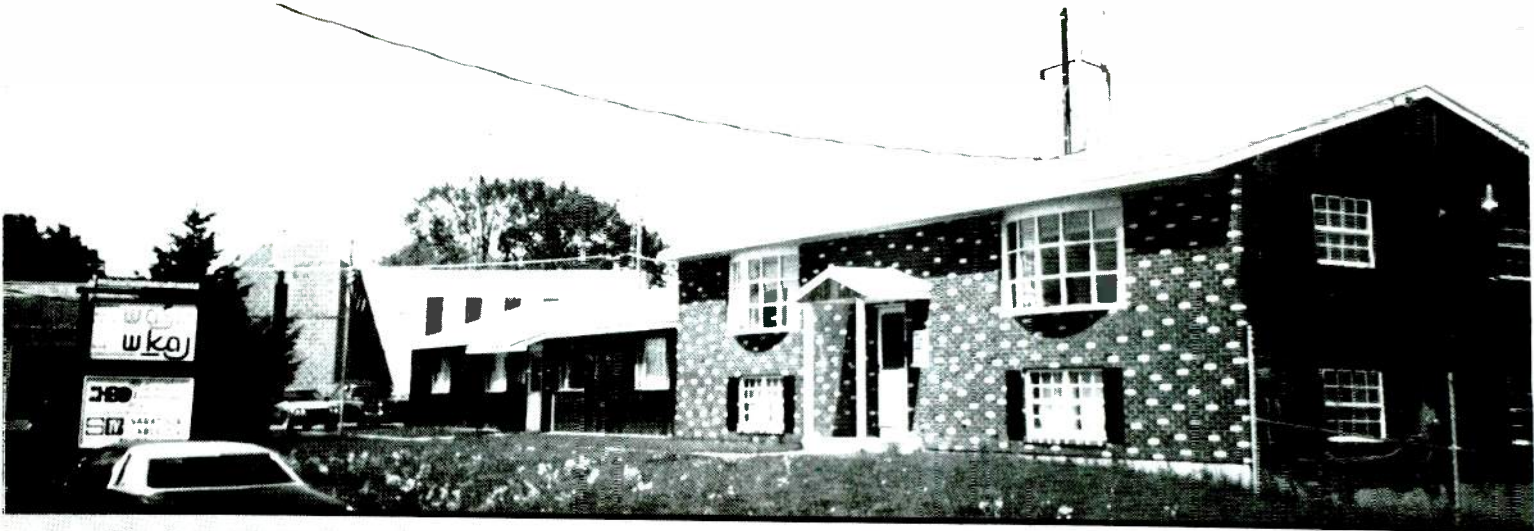
The Community Radio of Saratoga Springs, NY, facility. The AM and FM studios occupy the original 1-story building in the background. The new addition houses the cable operation.
