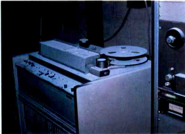
One of the remaining tape decks. Notice the amount of chemical on the deck.
