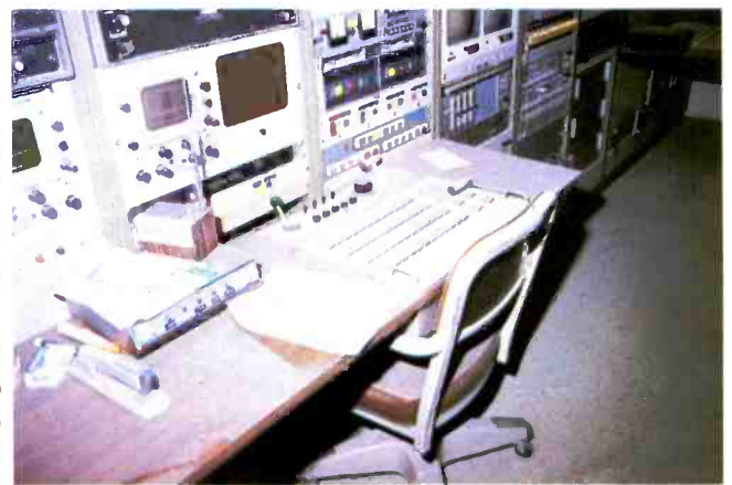
Master control. Note the dust from the fire extinguishers on the table. This can best be seen where the piece of paper has been moved.
