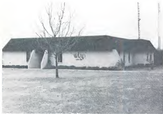
WLAP and WLAP-FM studio, office and transmitter building.
