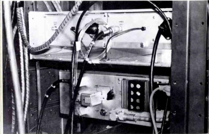
upper left photo shows the optic receiver mounted above the metallic cable remounted above the metallic cable receiver. The optic receiver was shown at the convention by Telemet. The lower left. It is shown the back side of the rack with pigtailed to cable splices. They are sped to the back edge of the chassis. It is so to courtesy of KSL-TV)
