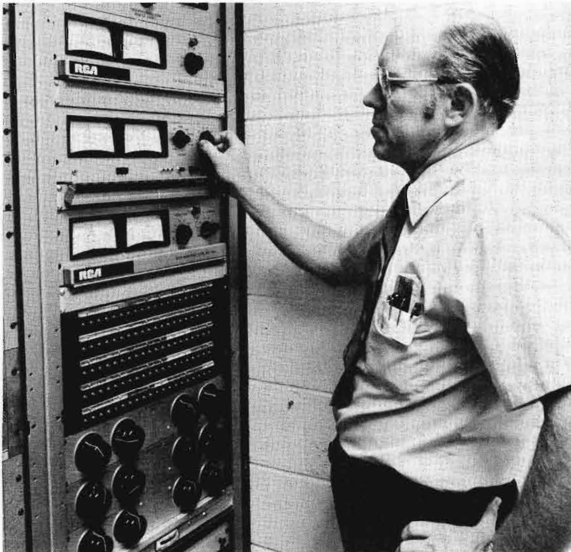
WDAI's maintenance supervisor, Harry Priester, examines a synchronous AM noise reading prior to performing the annual proof.
