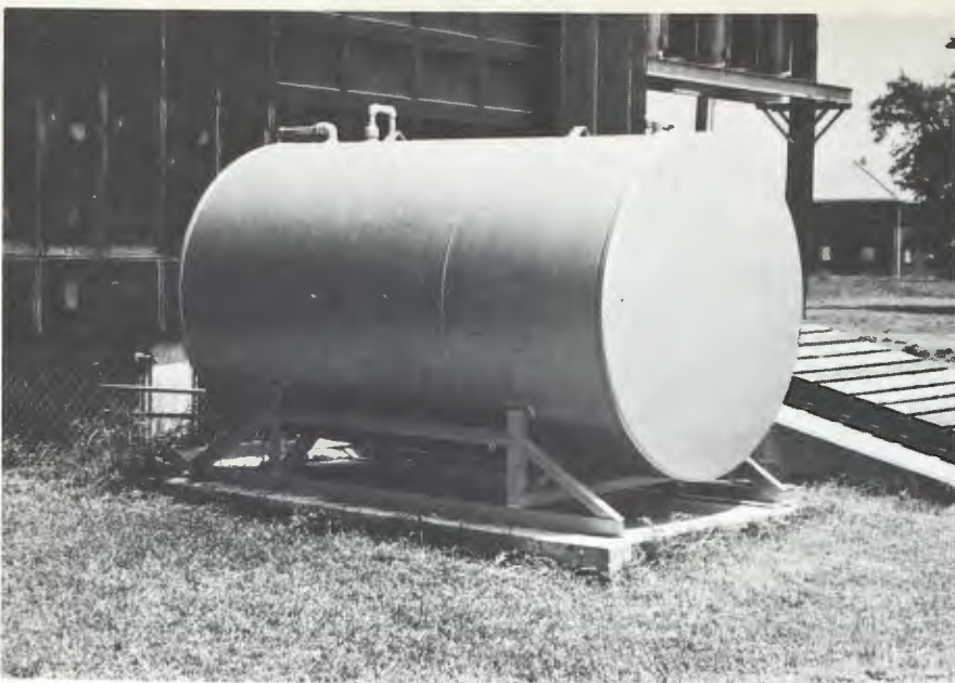
Fig. 2 Storms usually prevail from one direction. Locate the fuel tank on the opposite side of the building to provide protection.
