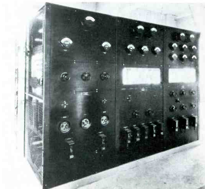
Fig. 5. The audio control bay of a five-kilowatt radio station. Circa 1929.
