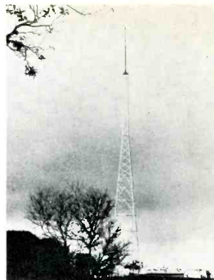
Six-bay turnstile antenna of Channel 7 in San Jose, Costa Rica, is on a 240' tower on a mountain 10,000' above sea level.
