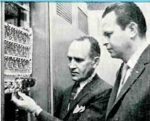
The control center of WDR-AM-FM is wired with Belden 8451 and 8700 miniature broadcast audio cables. Explaining the complexity of the installation to George Kyros is Orville J. Sather, Director of Engineering for WDR-AM-FM.
