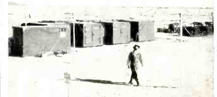
Fig. 4. The 50-kw VHF transmitter shelters.
