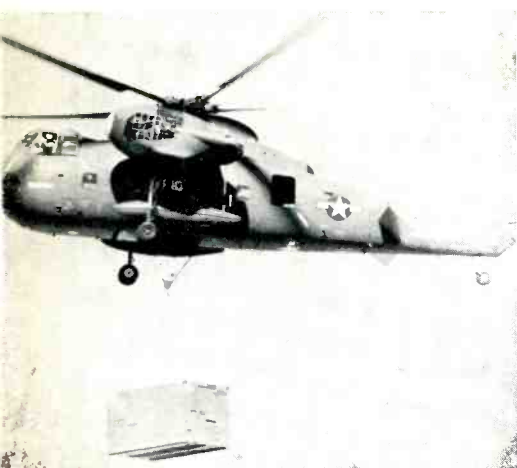
Fig. 1. Helicopter carries radio shelter.
