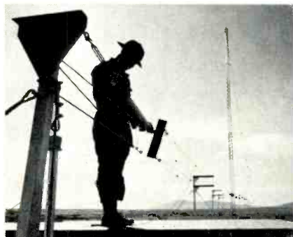
Fig. 5. GI tightens transmission line unit.
