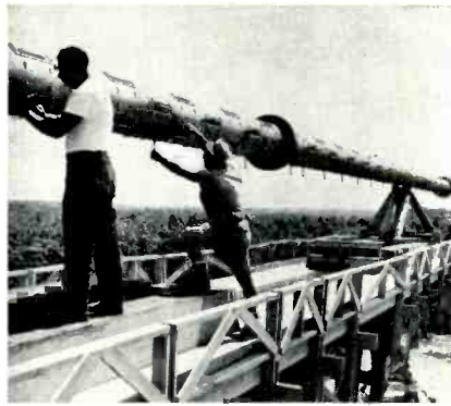
Fig. 4. Slotted cylinder UHF TV antenna.
