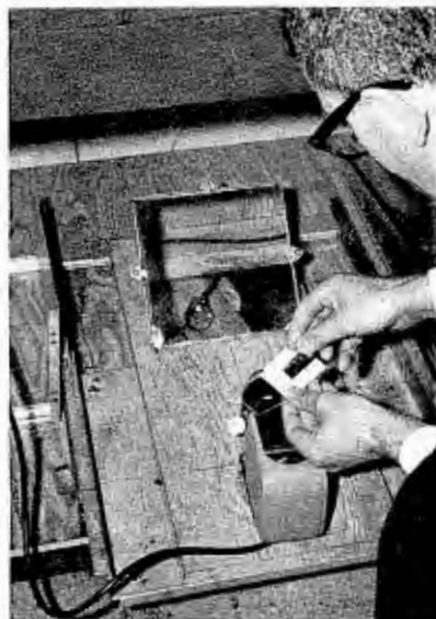
Fig. 2. Film clip is inserted into holder.
