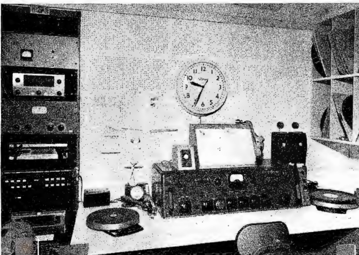
Fig. 1. WRFL No. 2 control booth; FM receivers are in rack at left.
