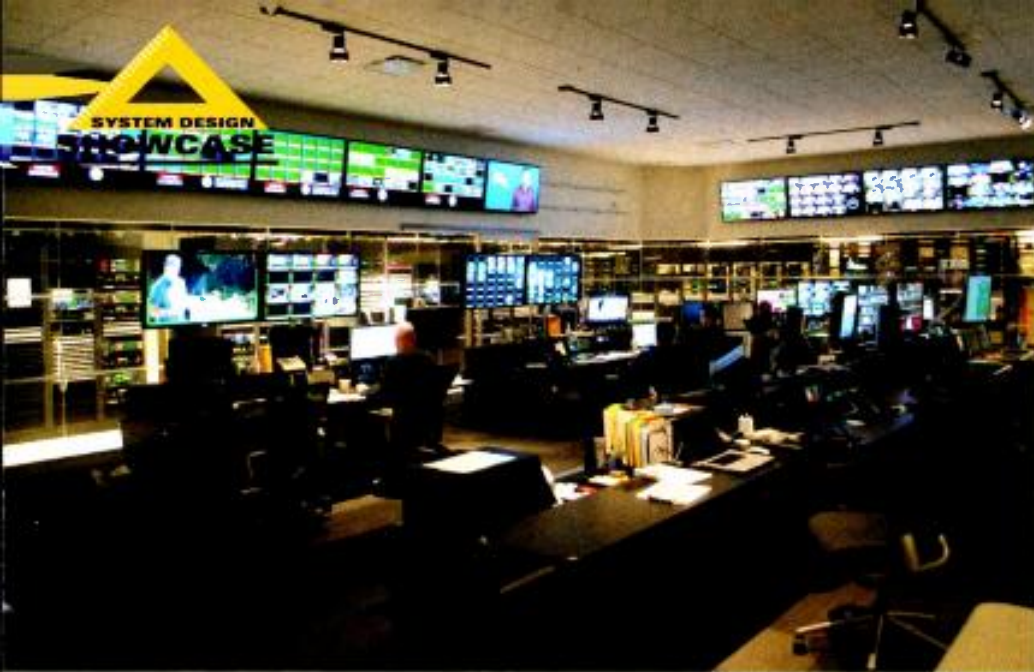
Shown here is the master control and transmission room. The transmission area employs a 512 x 512 EQX router to handle 132 incoming feeds, while an internal IP-based network allows signals to be monitored from any desktop in the building.
