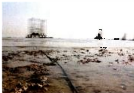
Here, fiber was run underwater out to man-made islands. The fibers each carried hundreds of channels of redundant audio and control channels for distribution of audio for PA systems, control for lighting fixtures, and video for projection and LED screens during Kuwait's 50 th Constitution Day Celebration.
