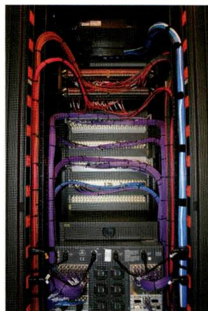
A Harris Platinum router (at bottom) ties the entire university news lab into the local PBS station WUFT infrastructure.
