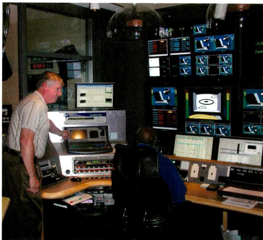
Senior project manager Bob Peck monitors operations in the Turner Network master control center, which employs NVISION's NV5100MC multichannel master control system.
