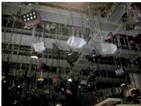
A lighting system supported by catwalks requires an extra 30lbs per sq ft in terms of load requirements.
