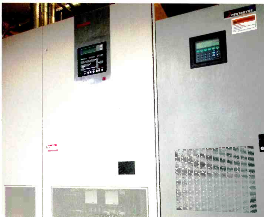
KTUD, VegasTV, in Las Vegas relies on a Toshiba G8000 UPS and a flywheel made by Pentadyne.
