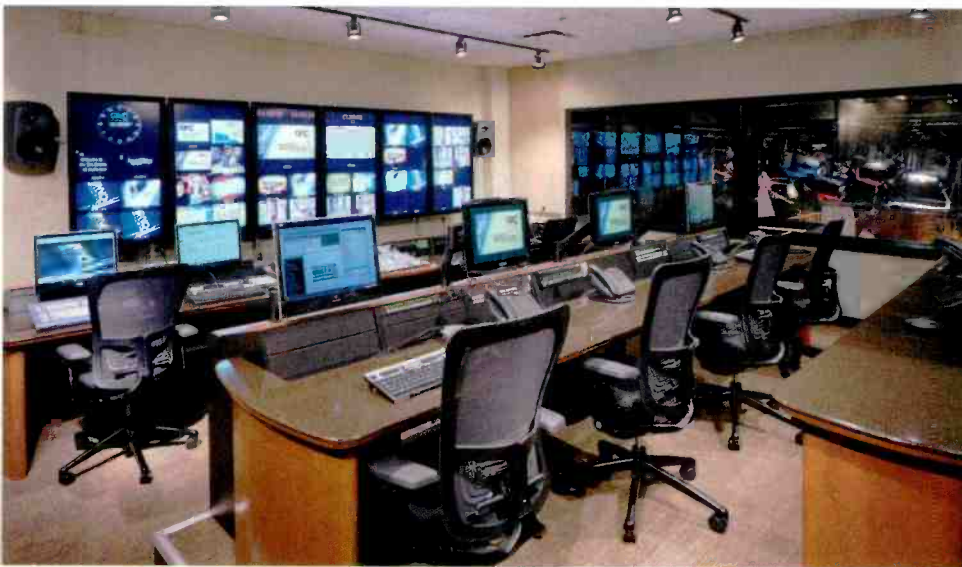
The main video control room has a Thomson Grass Valley Kayak 2.5 M/E switcher, Miranda Kaleido-X multi-image display, Chyron HyperX2 CG and RTS/Telex Cronus intercom.
