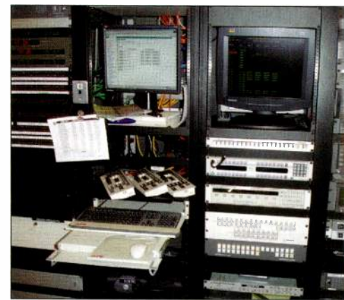
In the MC QC area, the AMX KVM switching system accesses the various control PCs, which configure the routers and UMD-type display system.
