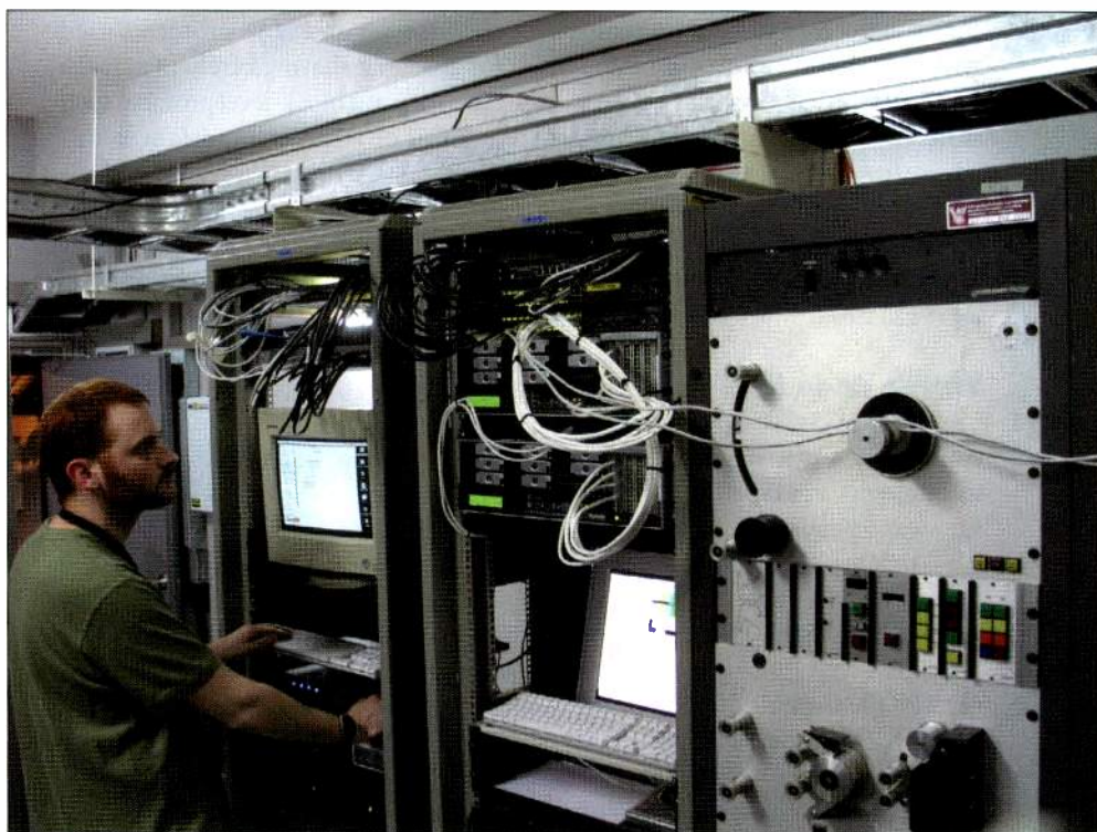
Studio Network Solutions' systems engineer Loring Weinkauff installs a globalSAN iSCSI initiator at Technicolor's Bangkok, Thailand, location.
