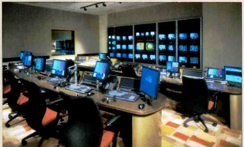
Food Network's multi-use control room is dedicated to the 7000sq ft main production studio. As part of the design, the director and TD can see and communicate with the program audio mixer through the small window to the far left.
