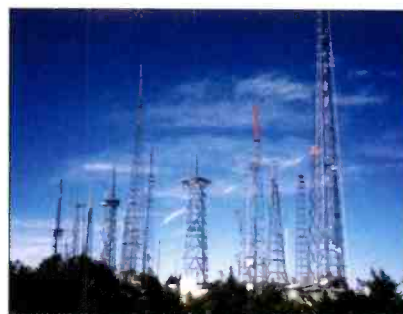
This view of Mt. Wilson antenna farm in Los Angeles was taken from the observatory visitor parking area in the spring of 2003. The far left tower is KCAL(TV) and the tower on the far right is KCET(TV). Photo courtesy Don Mussell.
