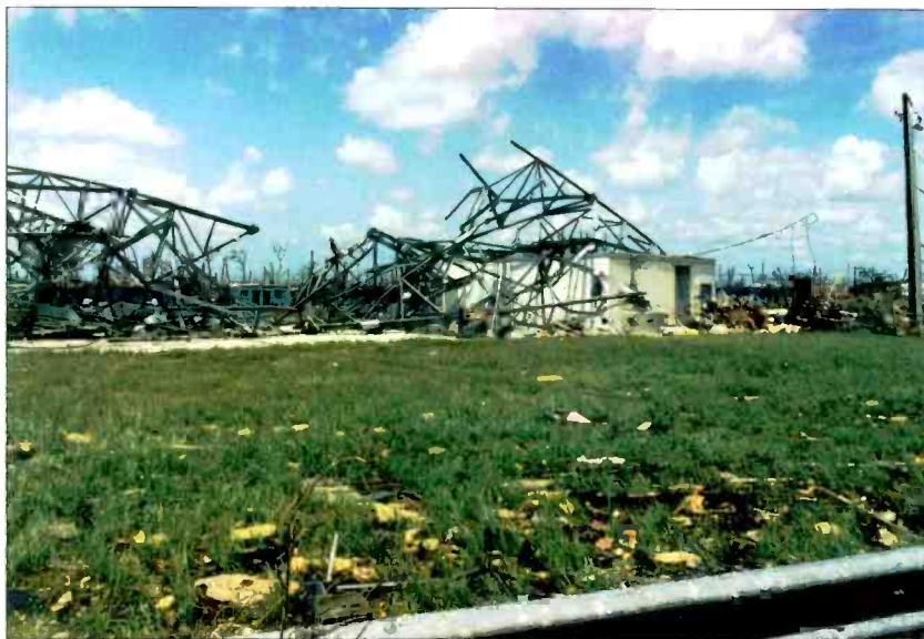
After a hurricane, a transmitting tower lies in ruins. You can't prevent such an event, but you can and should plan to recover from one.
