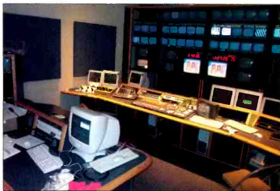
WALA's production control room features an Ikegami monitor wall with Evertz quad-splits. On the "Front Bench," from left to right, are the Vinten remote control for the Sony BVP-950 studio cameras, a Thomson Grass Valley Zodiac switcher and a Chyron Duet graphics station.
