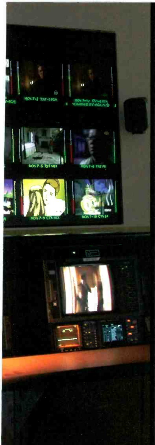
The transmissions operation center is divided into two portions: incoming and outgoing, the latter of which is pictured here. This area serves as a final QC point as signals from all 19 networks are sent out of the building to the satellite.
