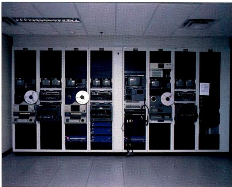
The central tape area of the media operations center features a variety of tape machines, including the "guard source VTRs," which provide a third level of on-air redundancy for high-profile programs.
