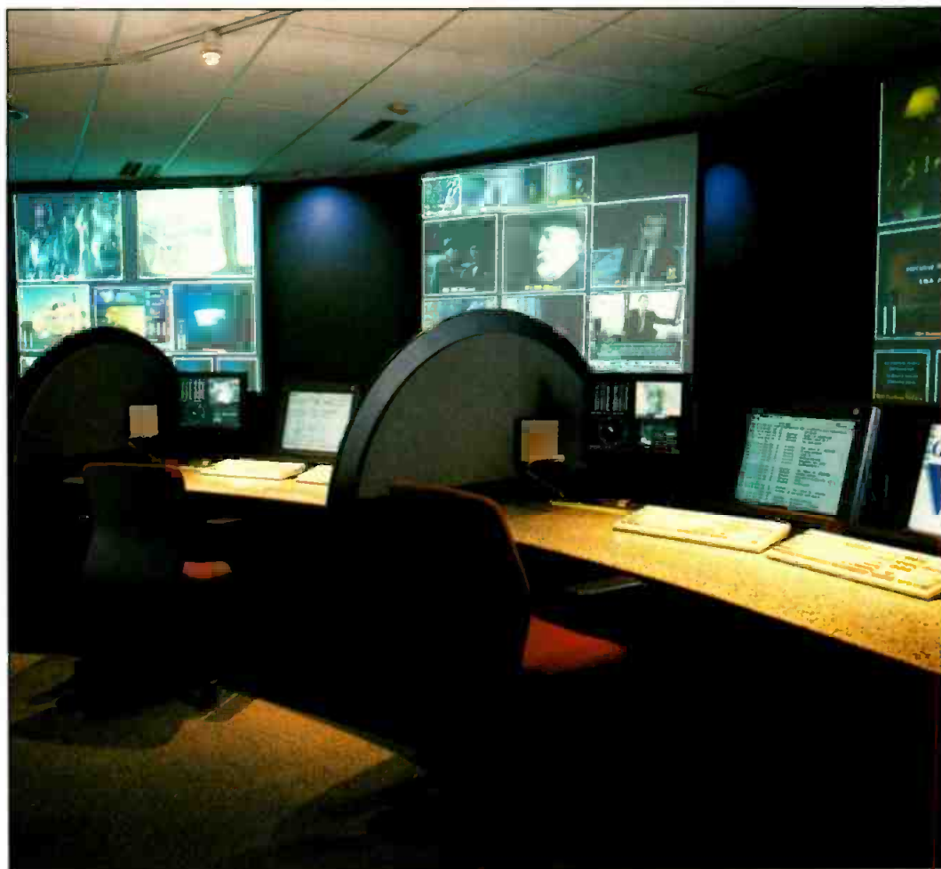
In the master control facility at GWNS' Harbor facility, above, each operator can customize the projection screen layout in order to efficiently monitor four networks.
