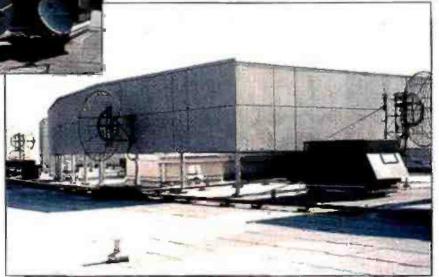
The roof is also an important part of the facility, with antennas for the STLs, RPUs and satellites.
