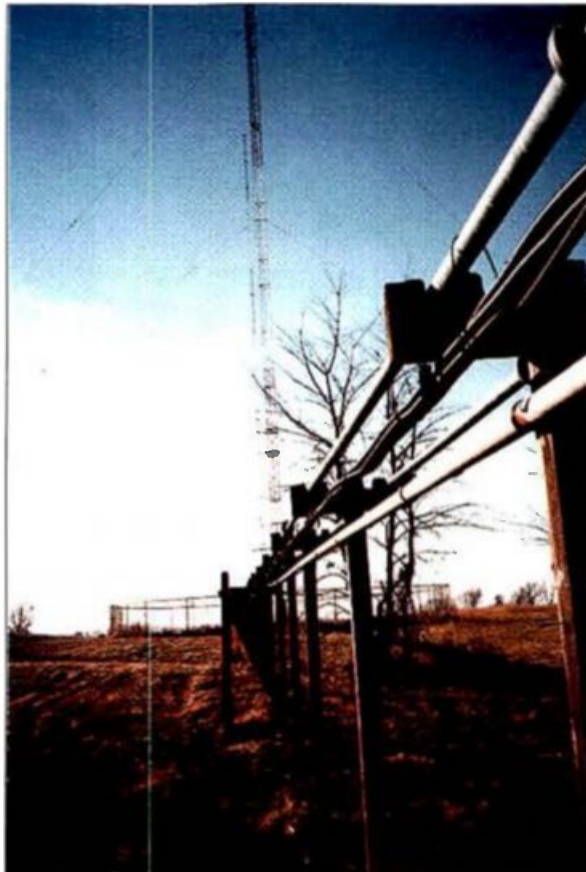
Feedlines and sampling lines must be maintained. Any line replacement must be made with an identical piece or the monitor sample calibration will be wrong.
