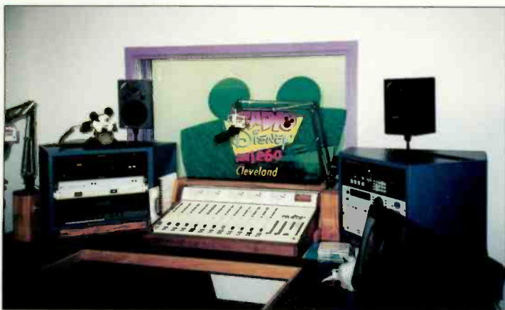
Some group owners rely almost entirely on contract engineers to build a studio, as was the case with this Radio Disney studio in Cleveland.
