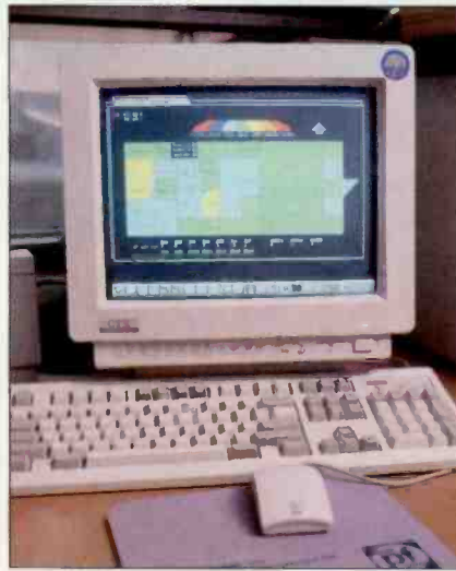
A PC monitors the HVAC system at the WCSX/WRIF facility in Detroit.
