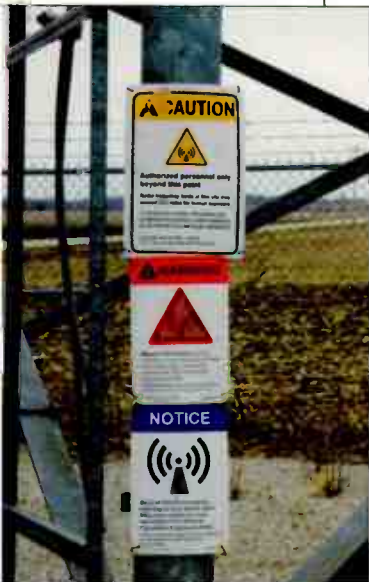
An example of improper sign placement.
