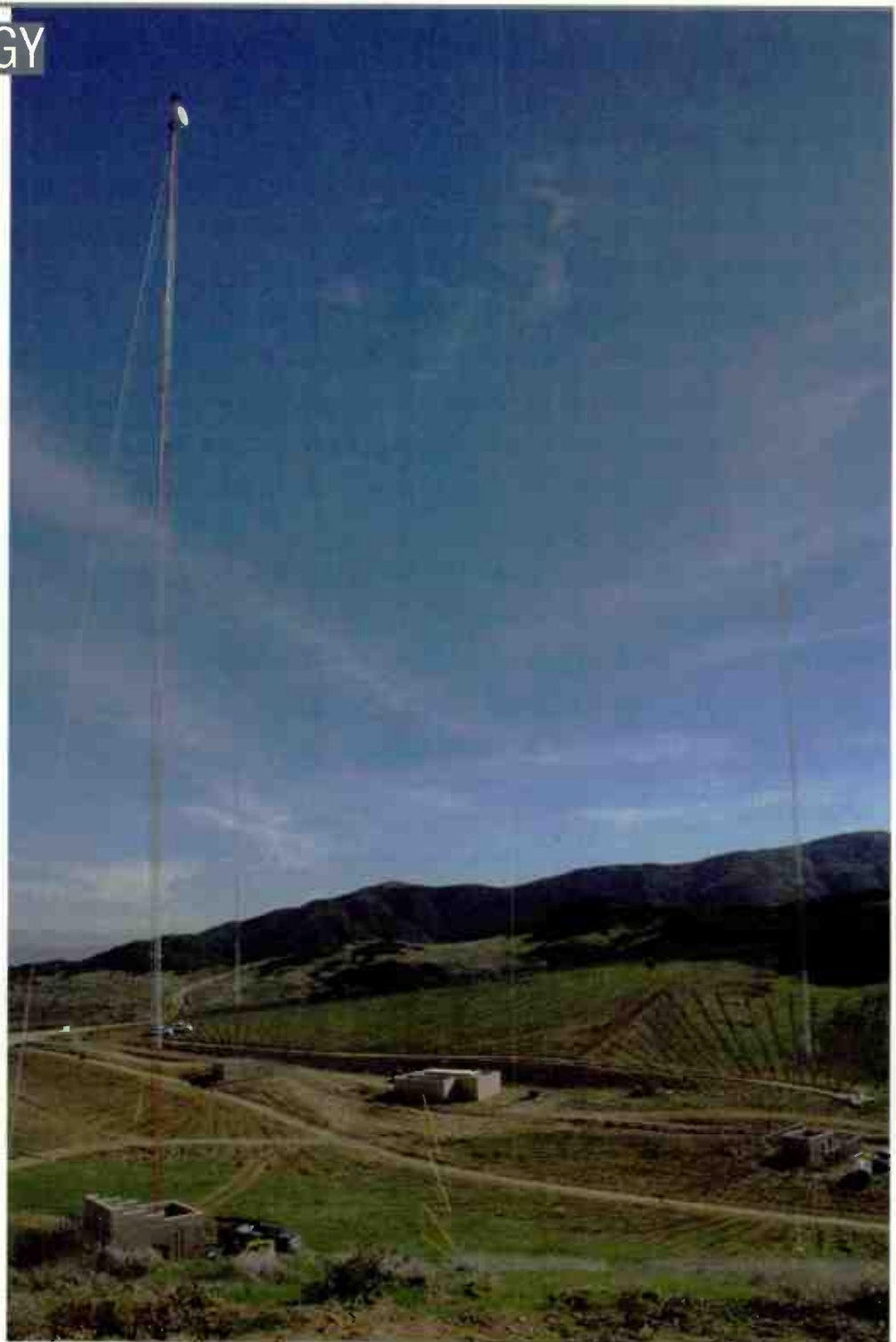
Above: KBRT AM740's tower array in California. Photo by Scott Fybush.
