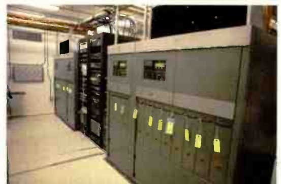
Right: Main and backup transmitters for both KRKO and KKXA.
