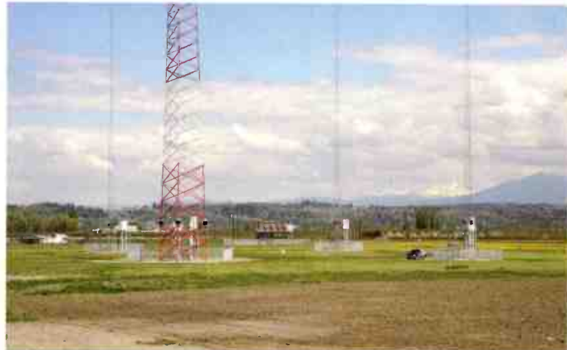
An extensive amount of time and effort was put in to protecting the KRKO/KKXA transmitter site from potential flooding.
