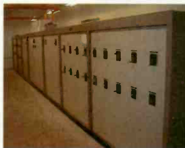
CUSTOM PHASOR INSTALLATION
