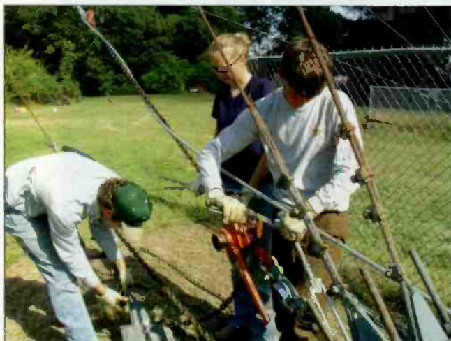
Pegasus Tower replacing the tower's guy wires.
