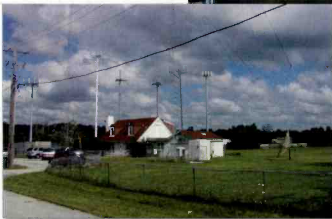
This radio station has a row of nearby detuned wireless towers. With regular maintenance to the detuning networks, this directional array remains stable.
