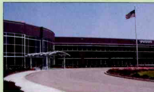
The 165,000 sq. ft. Harris Broadcast Headquarters houses Harris' Advanced Digital Engineering Center.
