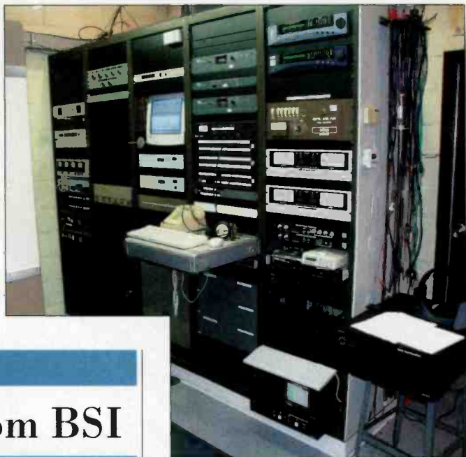
The racks at the WOR transmitter site. The IBOC exciter is mounted at the bottom of the rack on the right.
