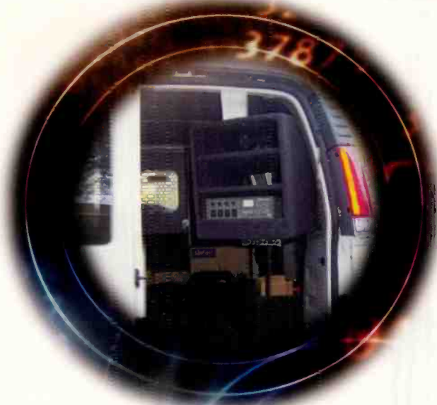
This cabinet is mounted off the floor of the Chevy Express van used for KFFN-AM. This mount provides clear floor space for stowing heavier materials.
