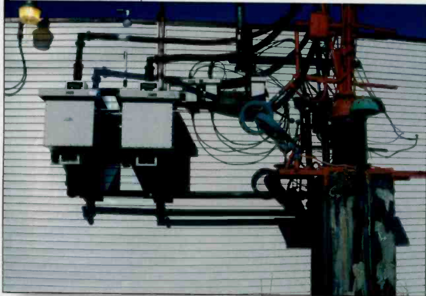
A thorough inspection of the tower and any accessory items must be done regularly. Photo by Jerry Goforth, WCLV-AM/FM.
